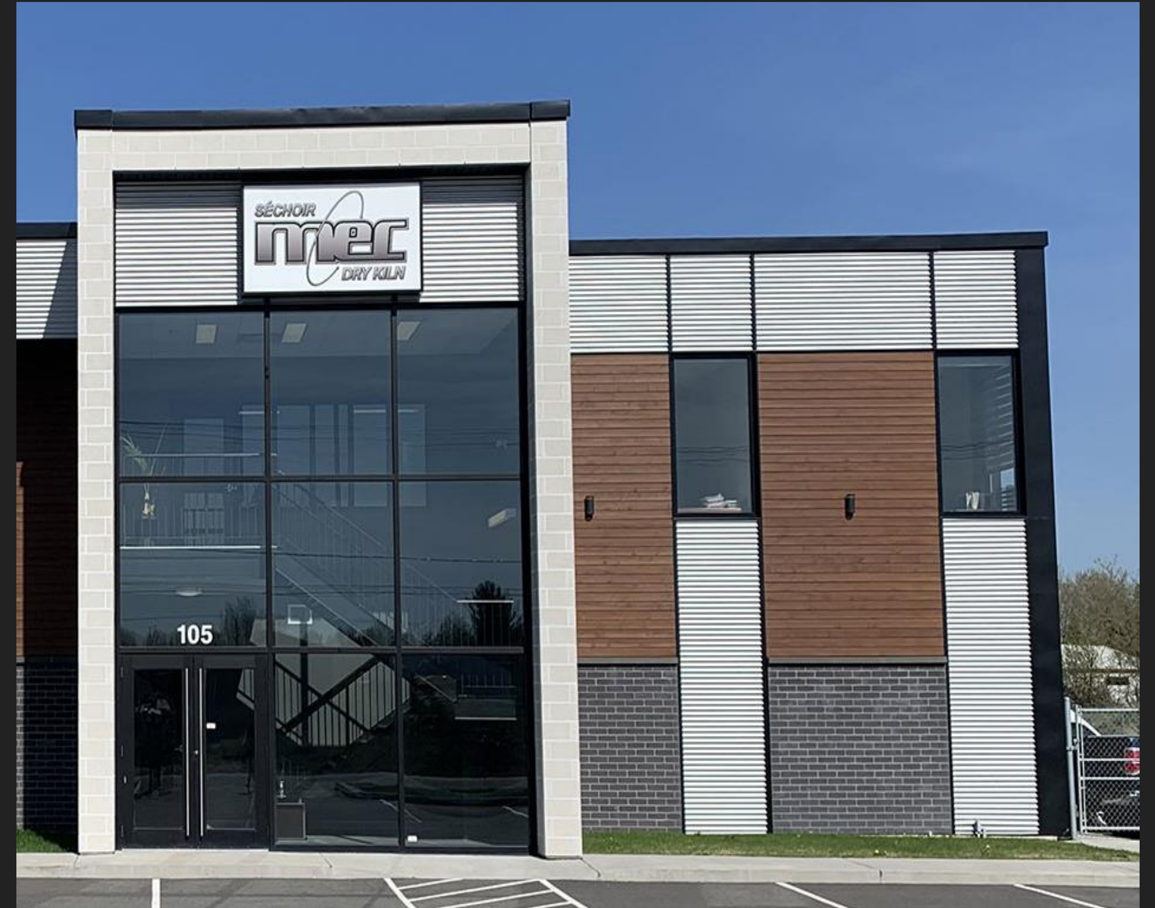
Séchoir Mec, division de Wellons Victoriaville, QC
